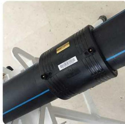
5- Place second pipe end up to first pipe push electrofusion coupler back onto the second pipe until the second marking area with bare hands after scraping and cleaning.
