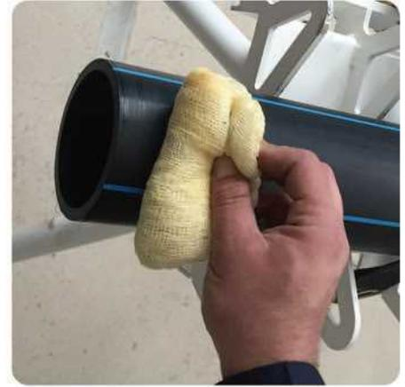
3- Clean pipe scraped area. Note: do not touch the scraped area with bare hands after scraping and cleaning.
