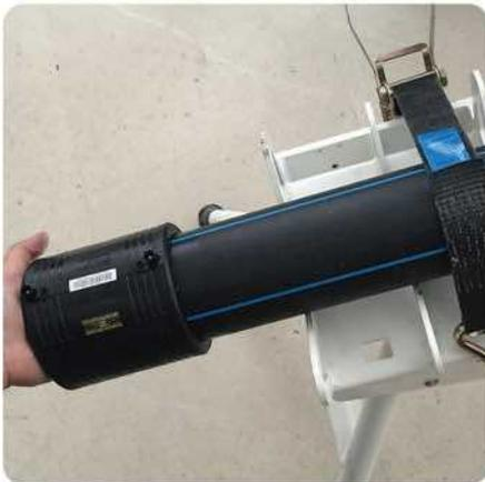
4- Insert pipe into electrofusion coupler.
