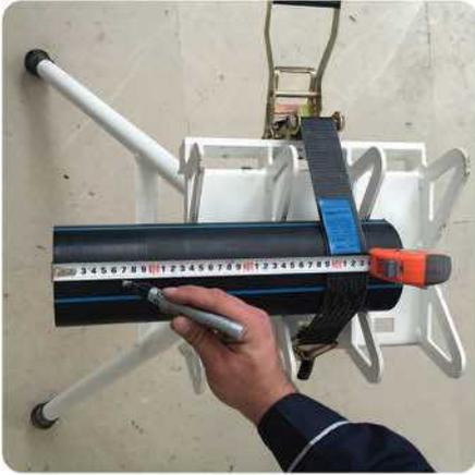
1- Measure area which has to be scraped with marker.
